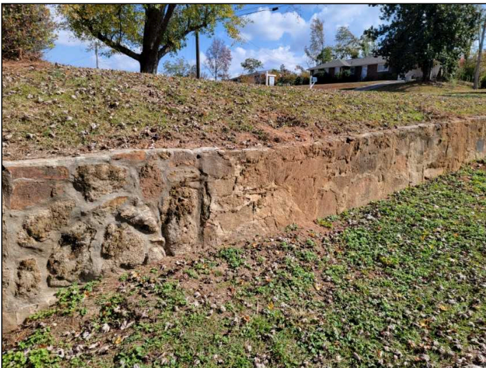
No Fall Protection
