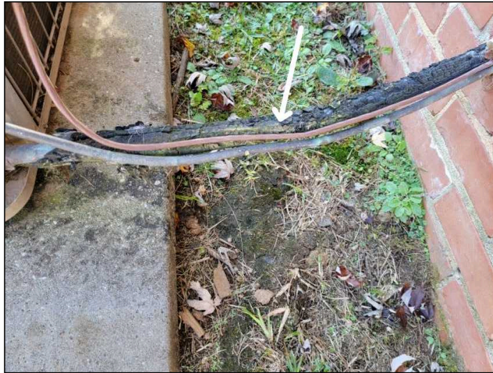
Missing/Damaged Insulation
