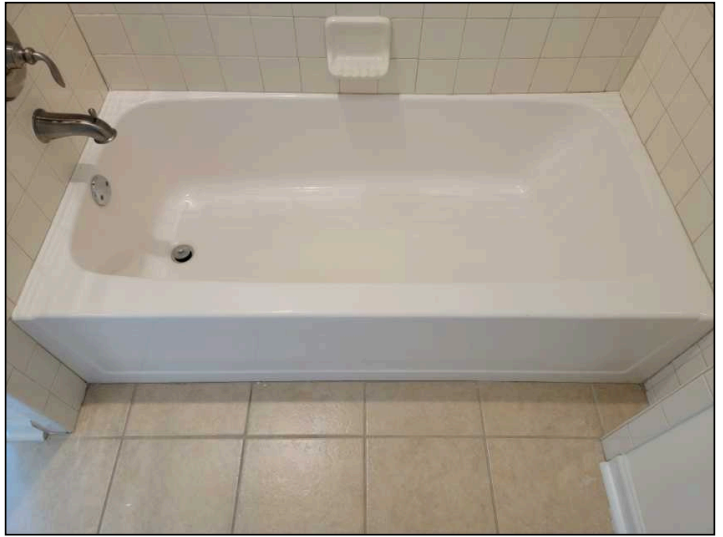
Caulk/Seal All Cracks & Gaps (Upstairs Guest)
