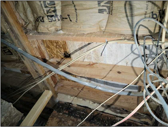
Missing Insulation
