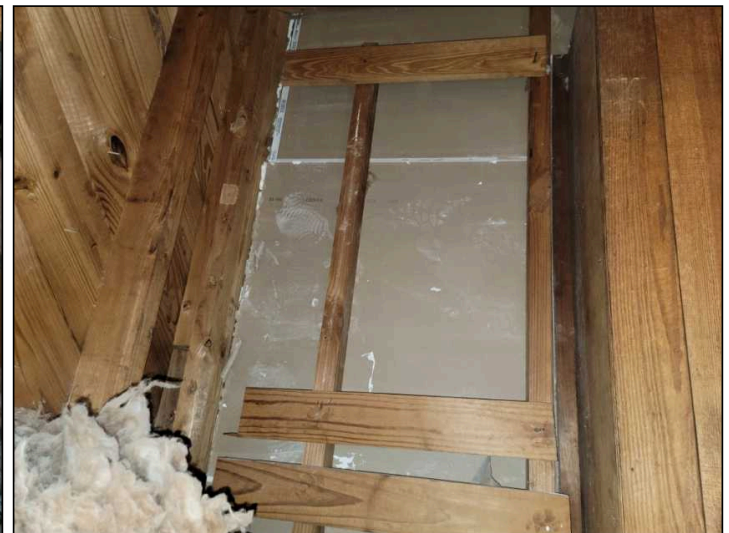
Sparse/Missing Insulation
