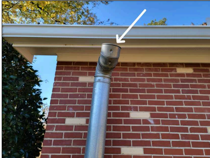
Open Vent/No Rain Cap
