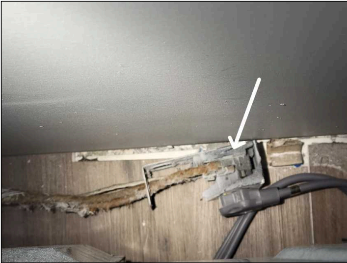
Range Plug Not Mounted/Missing Cover
