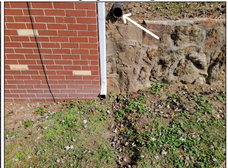
Open Drain Pipes
