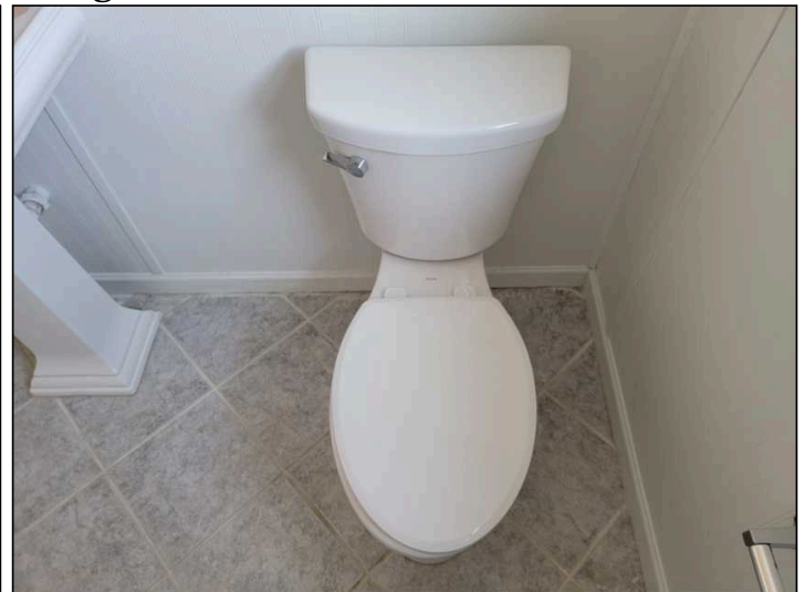
Loose Toilet (Guest)
